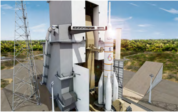
Fig. 3 – Partial retraction of the mobile gantry – Credit CNES
